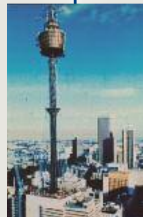
➔ 1975 – Sydney Tower – start of cable stay installation for this landmark which was the highest structure in the Southern Hemisphere when constructed. AUS
