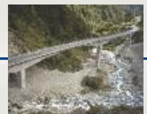
➔ 1999 – Otira Viaduct – balanced cantilever bridge built in the remote Southern Alps, New Zealand. NZ
