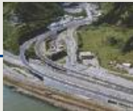
→ 1982 – Construction of twin-curved Ngauranga ‘flyover’ bridges in Wellington was carried out using the incremental launching method for the first time in Australasia and featured BBR post-tensioning. NZ
