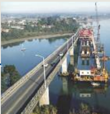
➔ 1972 – Upper Harbor Bridge – design input for bridge and balanced cantilever construction by BBRV in Zurich. The original bridge on the left and on the right, the 2004 ‘duplication bridge’ also constructed with BBR post-tensioning. NZ
