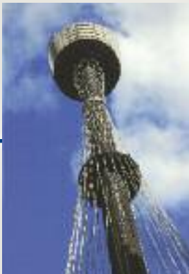
→ 1981 – Opening of Sydney Tower with its unique supporting net structure of BBR DINA stay cables. AUS
