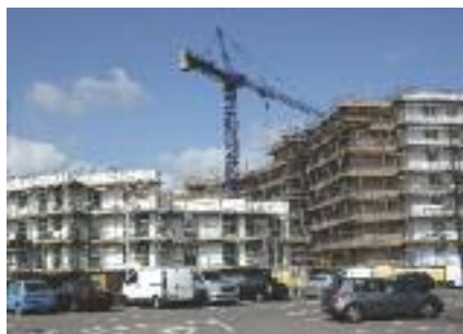
2 Bell Green residential development, Sydenham, UK
