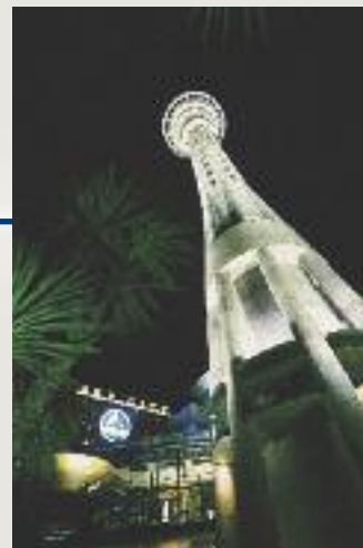
➔ 1995 – Sky Tower, Auckland, New Zealand – BBR Contech developed the BBR Multiwire Z36 internal anchorage which was the first time a BBR center stressing anchorage of this size had been used anywhere in the world. NZ
