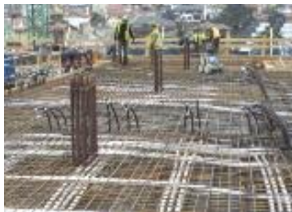
1 Marques de Valdecilla Hospital extension, Santander, Spain
