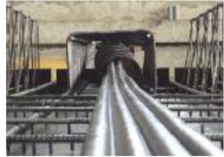
3 Car park, Warmbad Villach, Austria
