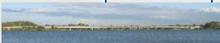
→ 1982 – Opening of the longest road bridge in Western Australia – Mount Henry Bridge, Perth which featured BBR post-tensioning. AUS
