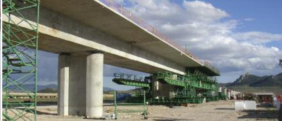
VIADUCTS IN VILLENA-SAX, SPAIN
