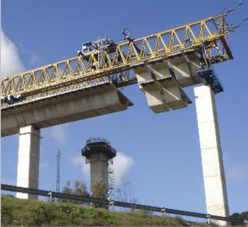
DESPEÑAPERROS VIADUCTS, SPAIN
