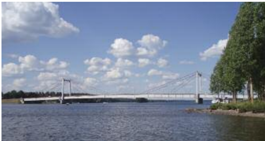
Dischinger's Strömsund Bridge in Sweden is celebrated as the first true cable-stayed bridge.
