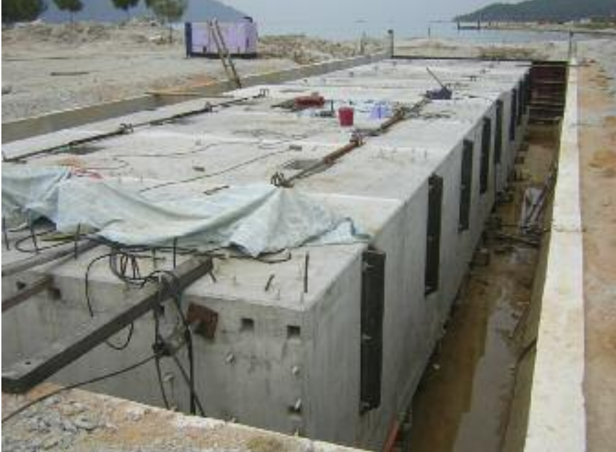
SEGMENTAL PONTOON, LUMUT PORT, PERAK, MALAYSIA
