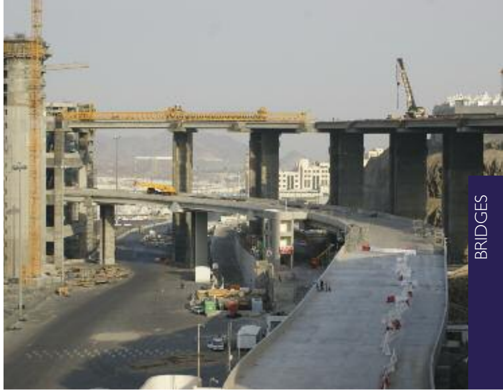
JAMARAT BRIDGE, SAUDI ARABIA
