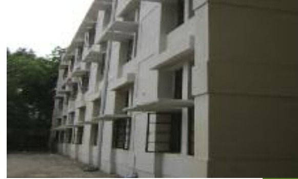
SEISMIC RETROFITTING OF SCHOOL, NEW DELHI, INDIA
