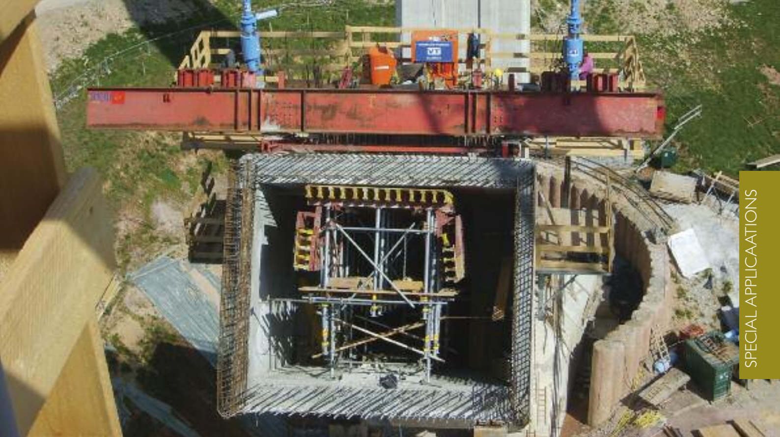
Arch cross-section, VT strands – elevator in the rear position during a lift procedure.
