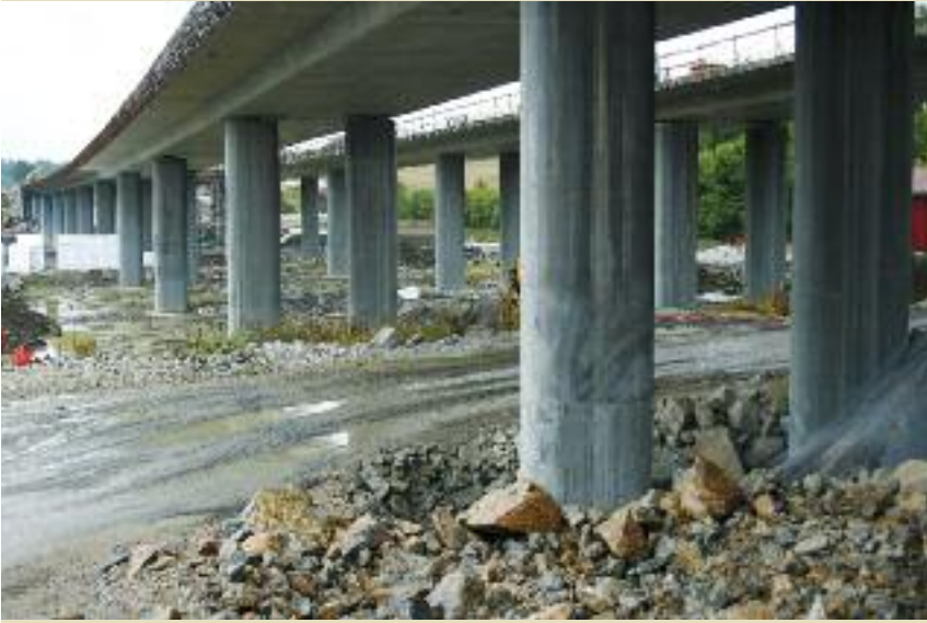
EI 8 MOTORWAY BRIDGES, LANGÅKER – BOMMESTAD, NORWAY
