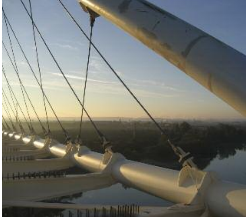
INSTALLATION OF LOCKED COIL ROPE STAYS, CÓRDOBA & ZARAGOZA, SPAIN
