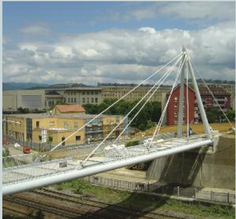
FORT HATRY RAILWAY BRIDGE, BELFORT, FRANCE
