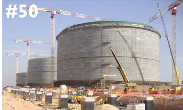
2012 – Ruwais Train LPG Storage, Abu Dhabi
