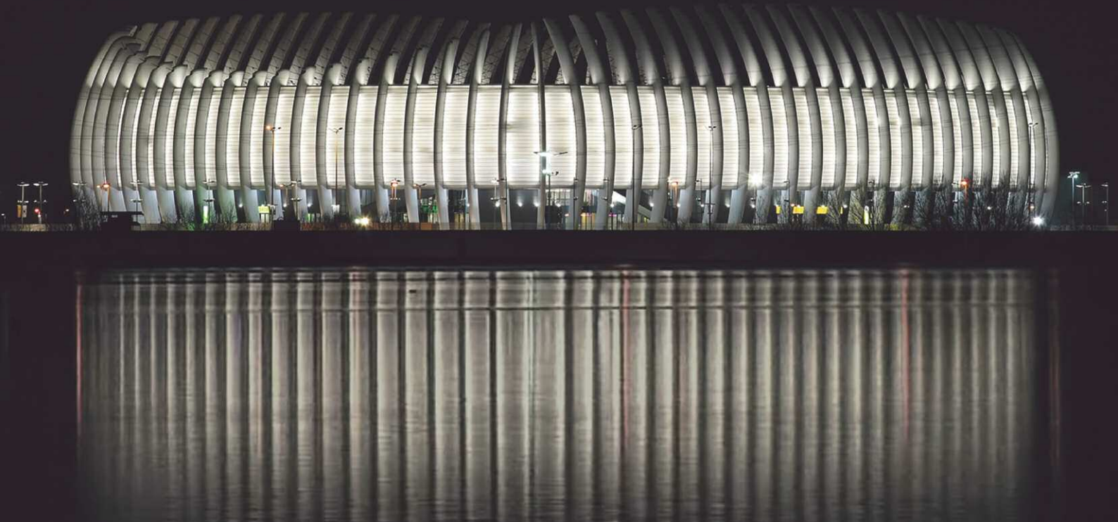
Kulmbachtal Bridge, Germany – BBRVT CONA CMB band
