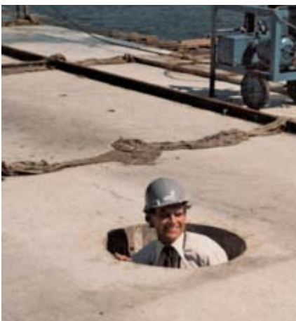
▲ 1970s: Josef Koch donned a hard hat to inspect work on Sterling Bridge in Perth, Australia.
